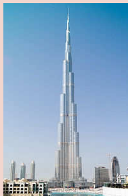
The Burj Khalifa, the tallest man-made structure in the world, opened in Dubai in January 2010.
